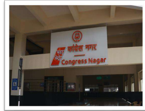
MAIN ENTRANCE OF CONGRESS NAGAR METRO STATION
