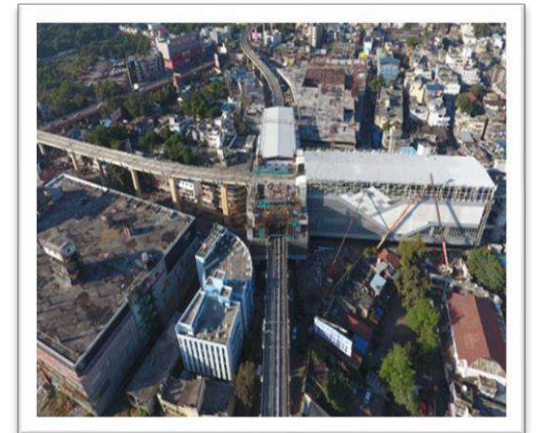
AERIAL VIEW OF SITABURDI INTERCHANGE METRO STATION
