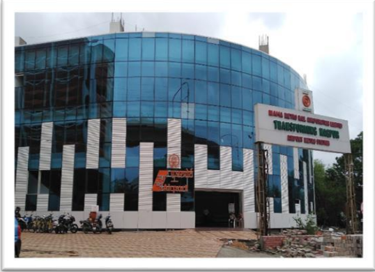
MAIN ENTRANCE OF AIRPORT METRO STATION
