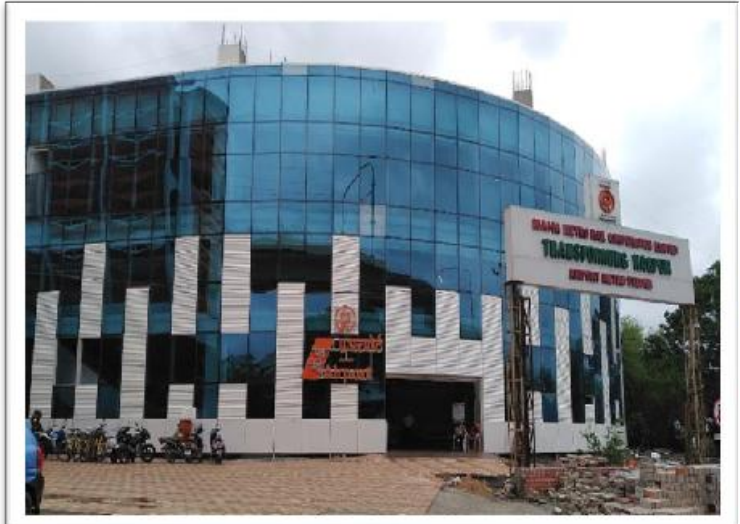
MAIN ENTRANCE OF AIRPORT METRO STATION
