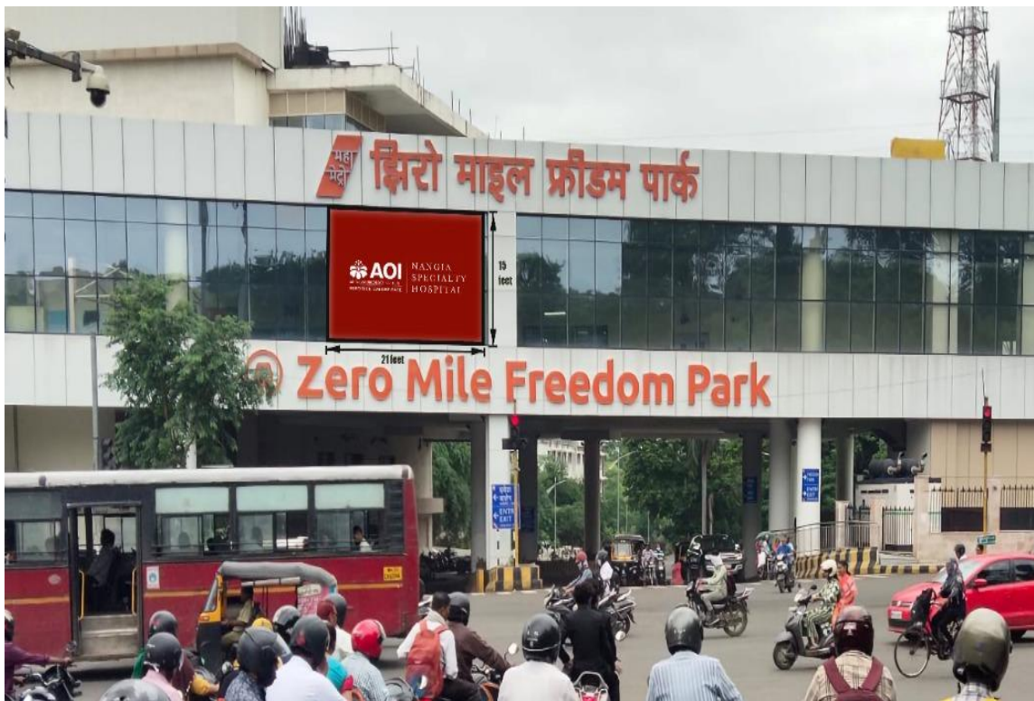
Zero Mile Metro Station
