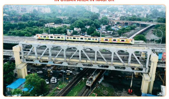
For the first time in the history of Indian Railways, 22 meter wide Double Decker Steel Girder was launched across railway track. Such a 4-layer transportation system is being constructed for the first time in the country. The structure weights 1670 MT and it is the heaviest Double Decker Steel over Railway Tracks in an urban area.
