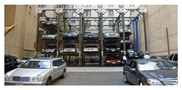
Figure 20 Multi-level stack parking NYC
