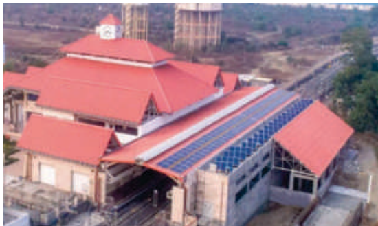
Solar Panels at Khapri Metro Station
