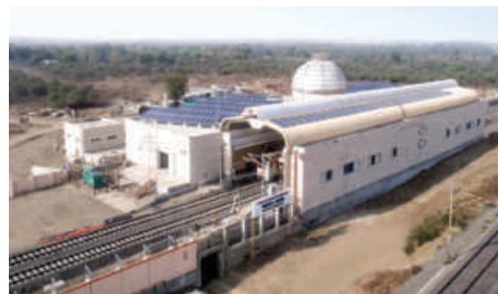
Solar Panels at New Airport Metro Station
