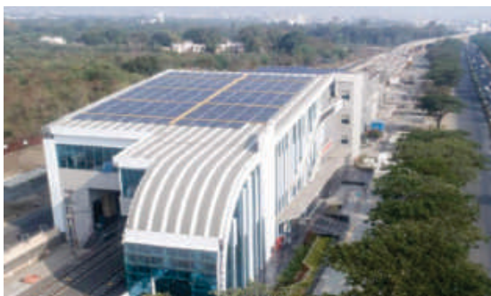
Solar Panels at Airport South Metro Station
