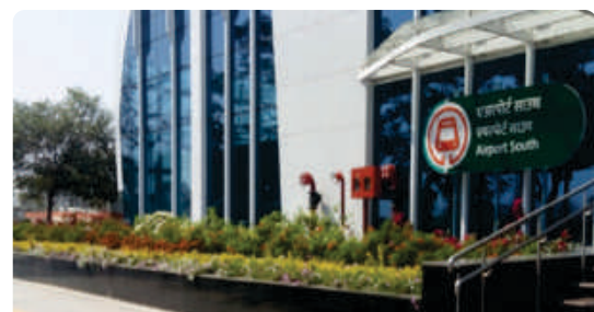
Landscaping at Airport South Metro Station
