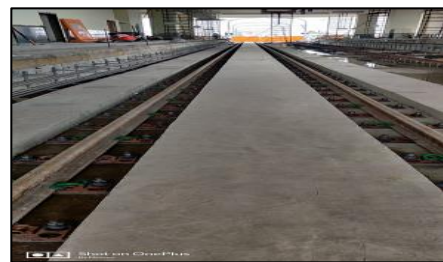
Finished MSS Floating Track Slab
