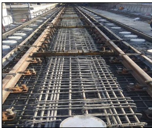
Reinforcement of MSS Track Slab
