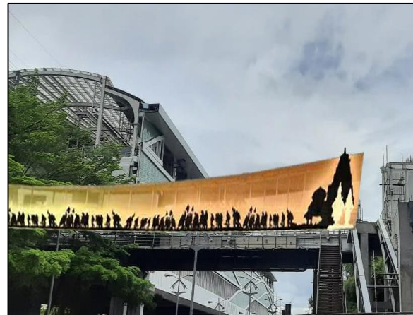
Warkari Theme at Sant Tukaram Nagar Station
