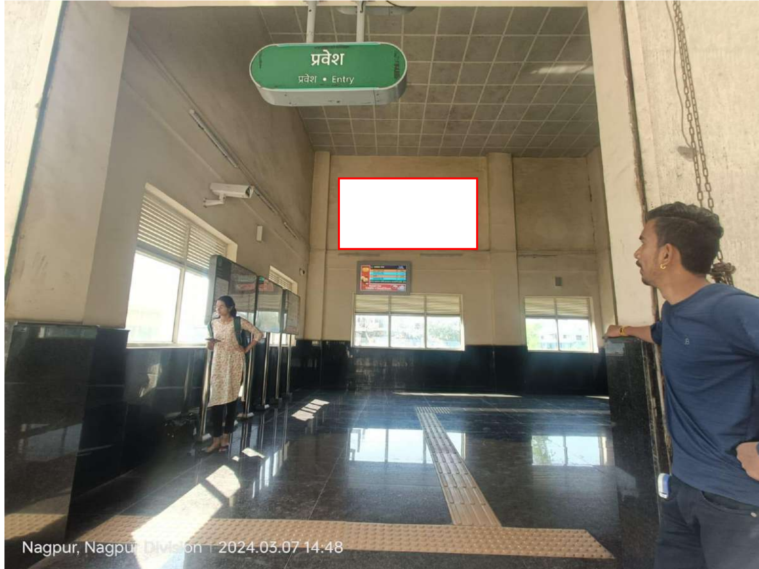
Ujjwal nagar metro station entry rights side road Wall 8x5
