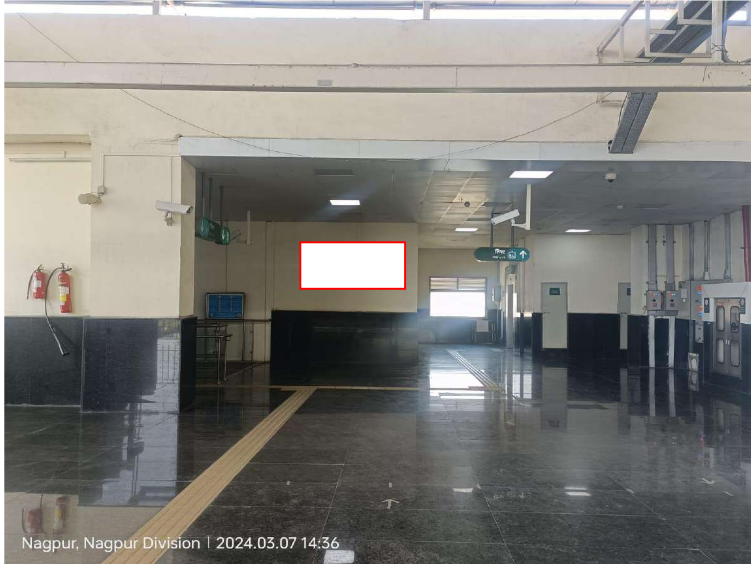
Ujjwal nagar metro station platform 2 exit Wall 8x5
