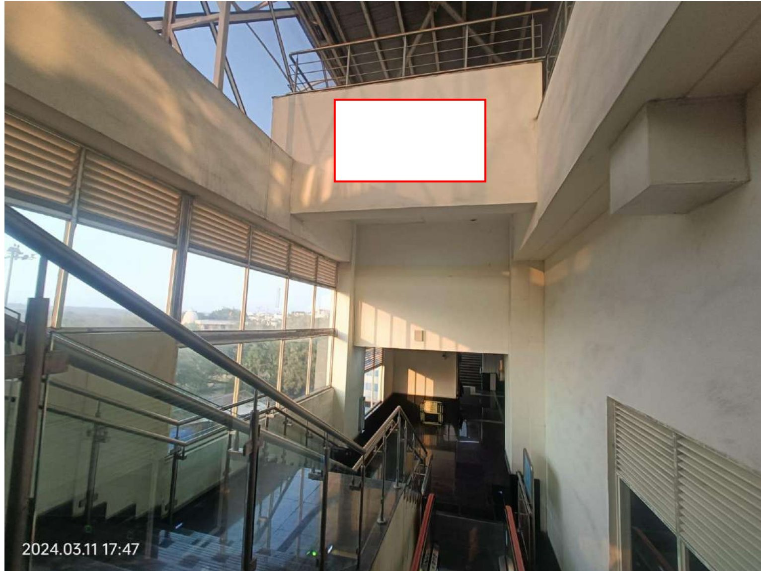
Vasudev nagar metro station platform 1 escalator upper Wall 8x5
