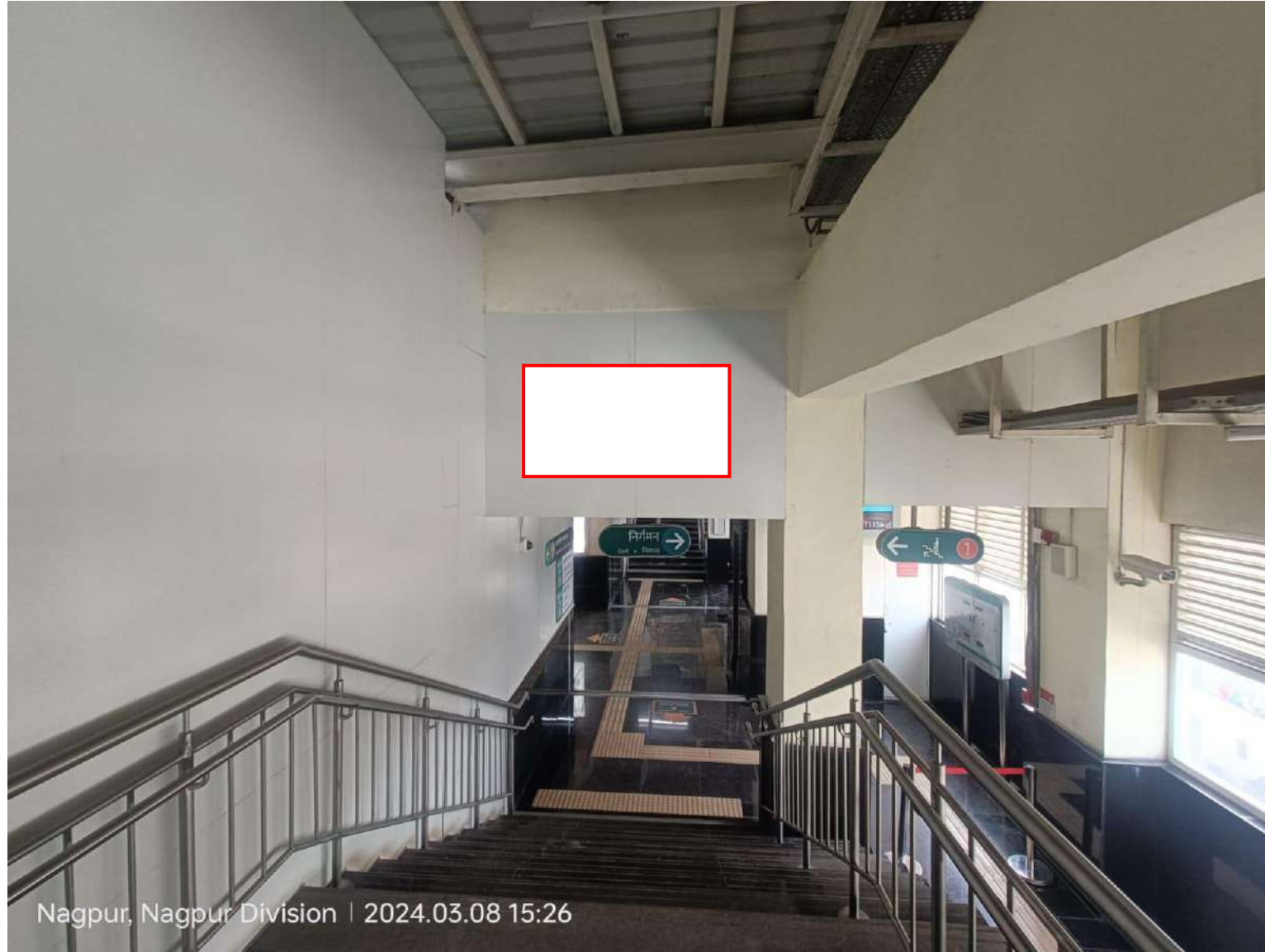
Nari metro station platform 1 staircase upper Wall 8x5
