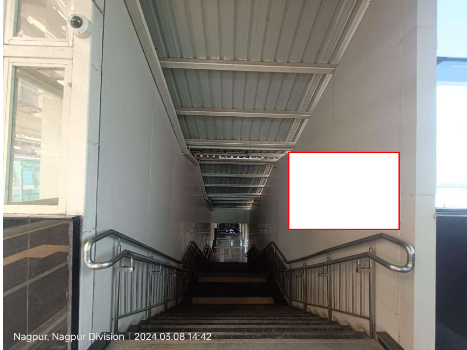
Gaddigodam sqr metro station platform 2 staircase side wall 8x5
