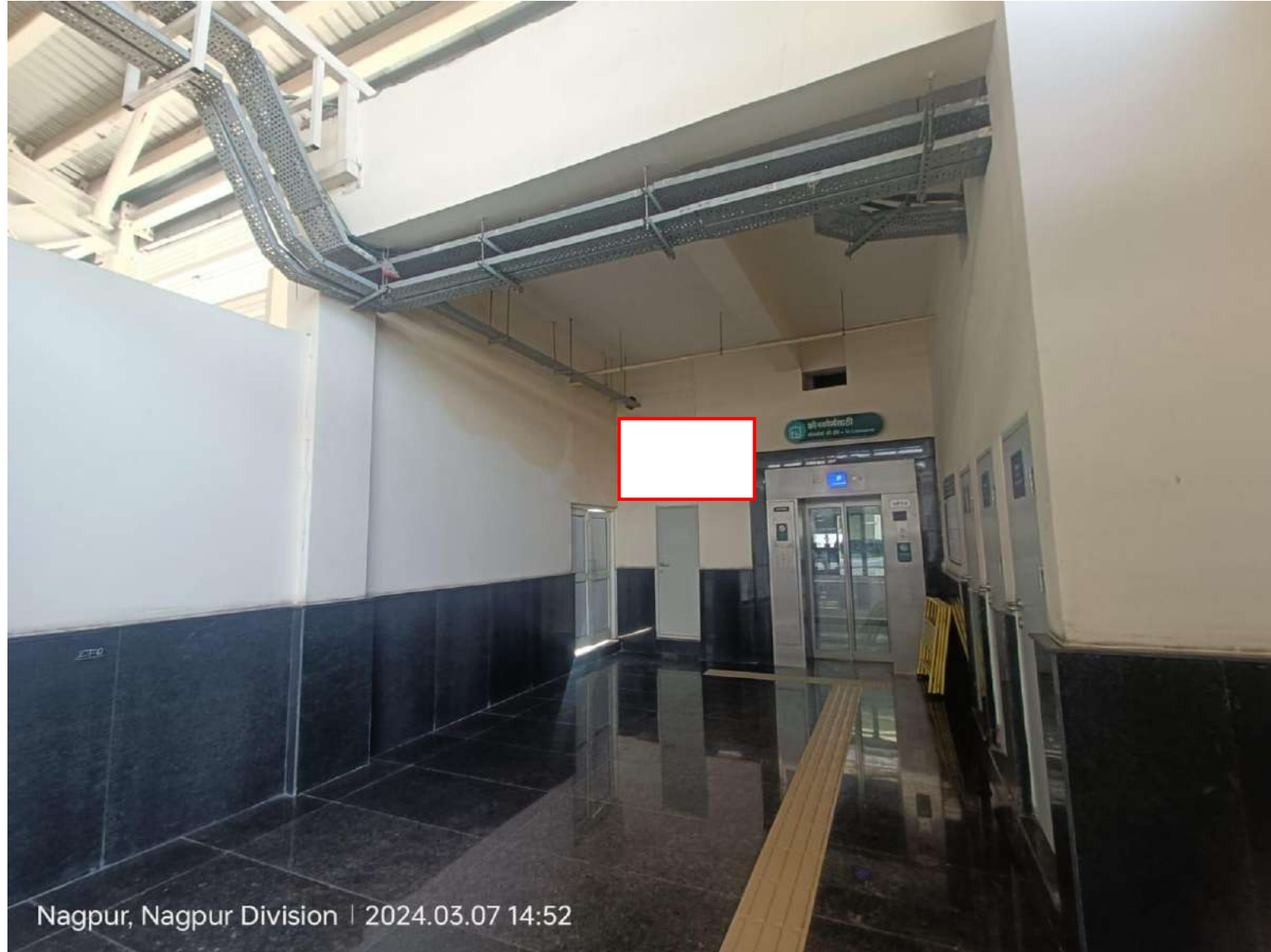
Ujjwal nagar metro station platform 1 lift 3 wall 8x5
