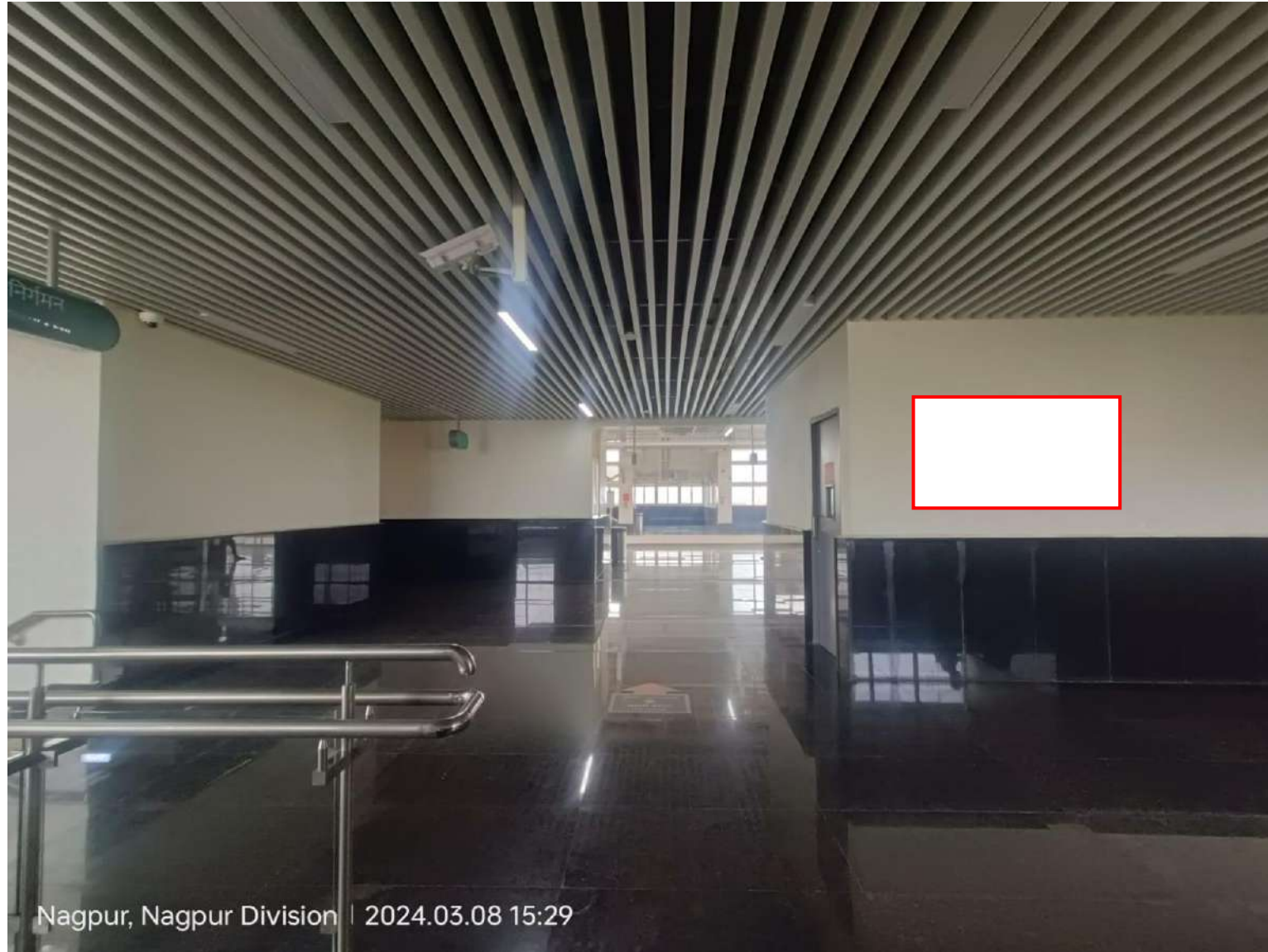
Nari metro station platform 2 entry wall 8x5
