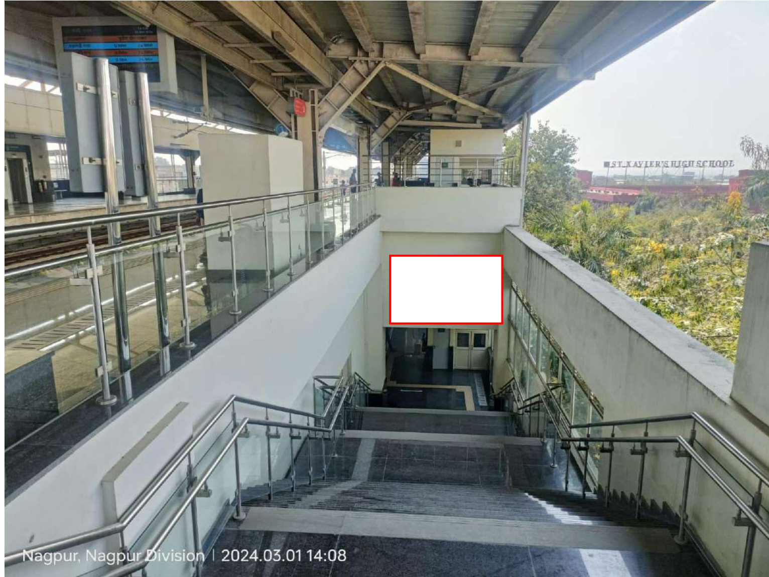
Bansi Nagar metro station platform 1 staircase gantry 8x5
