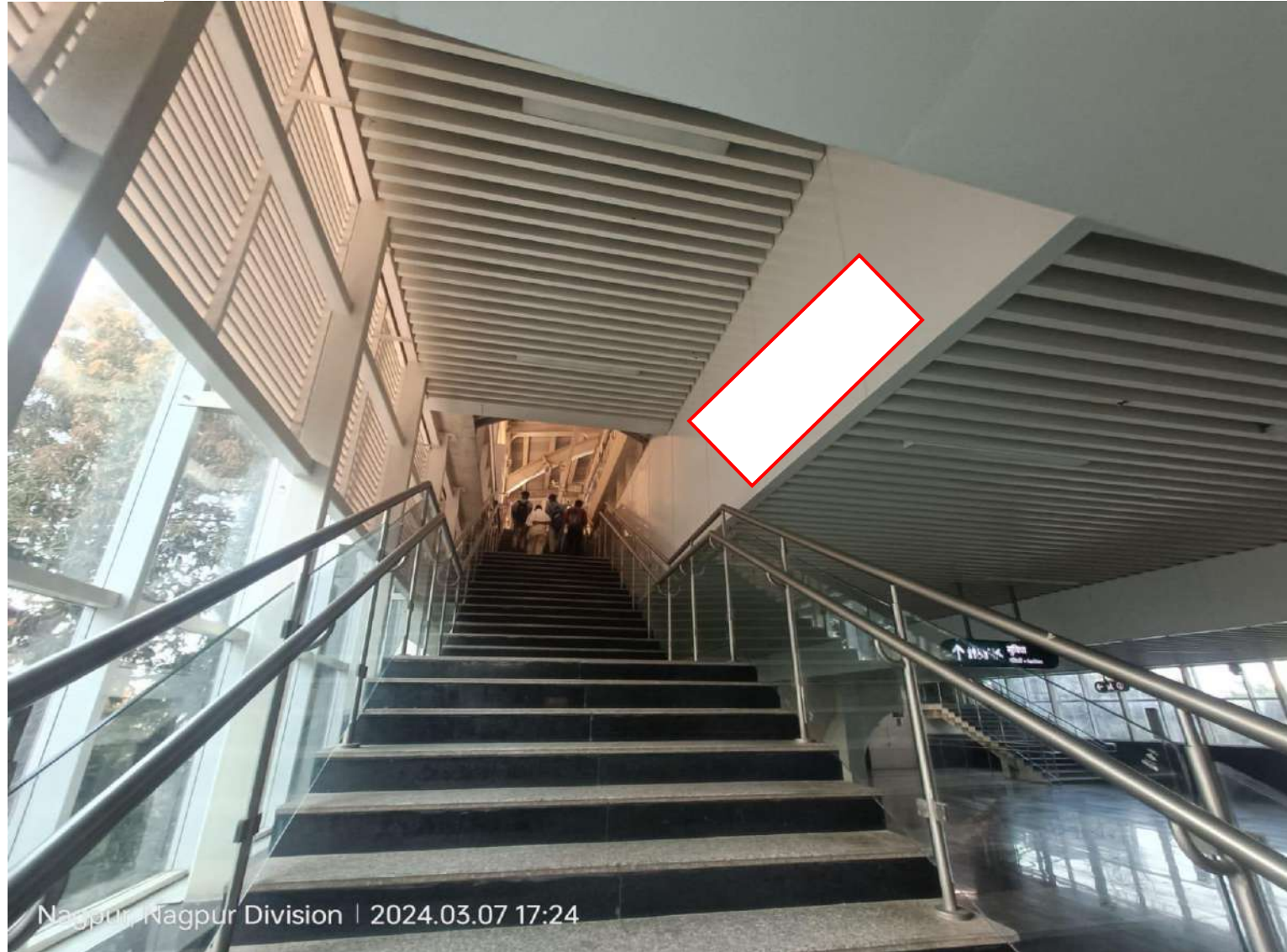
Congress nagar metro station platform 1 staircase side wall 8x5
