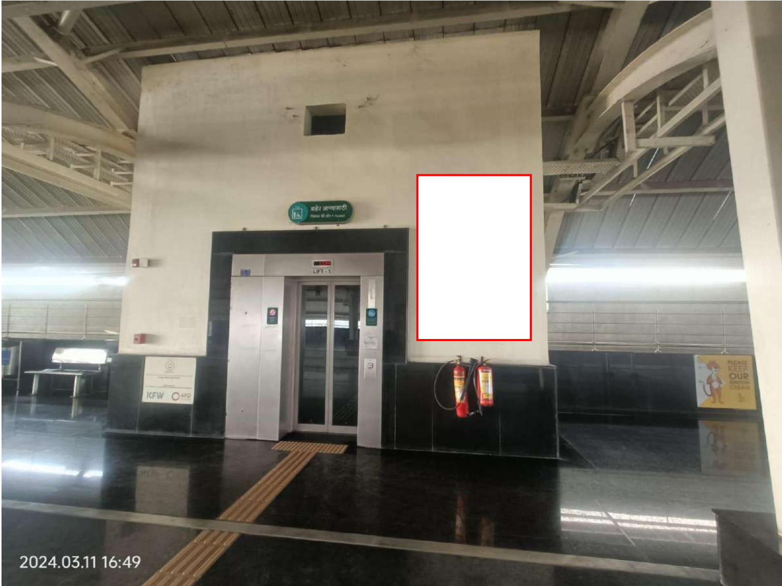
Subash nagar metro station platform 1 lift 1 right side wall 5x8
