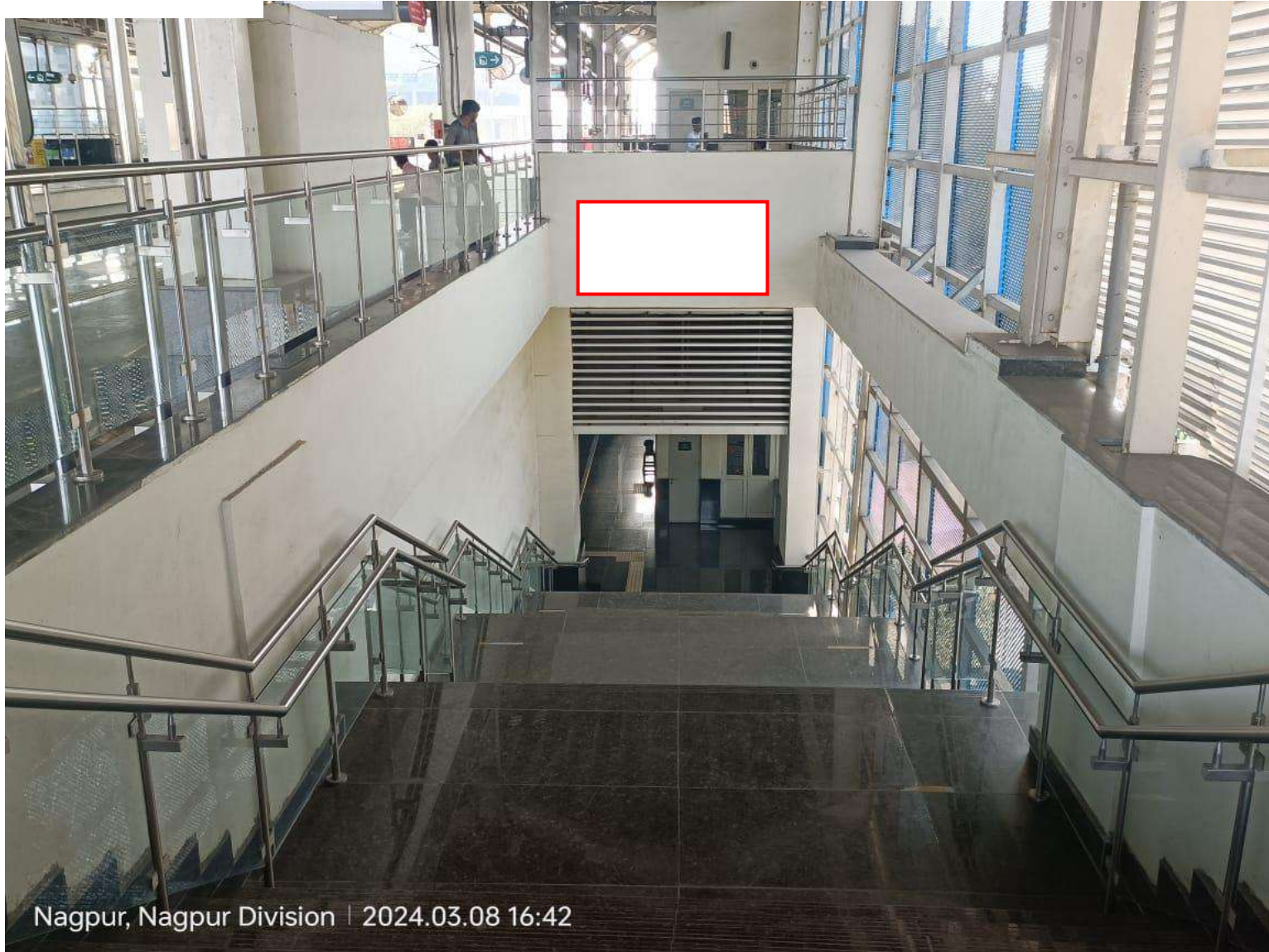
Institution of engineers metro station platform 1 staircase upper Wall 8x5
