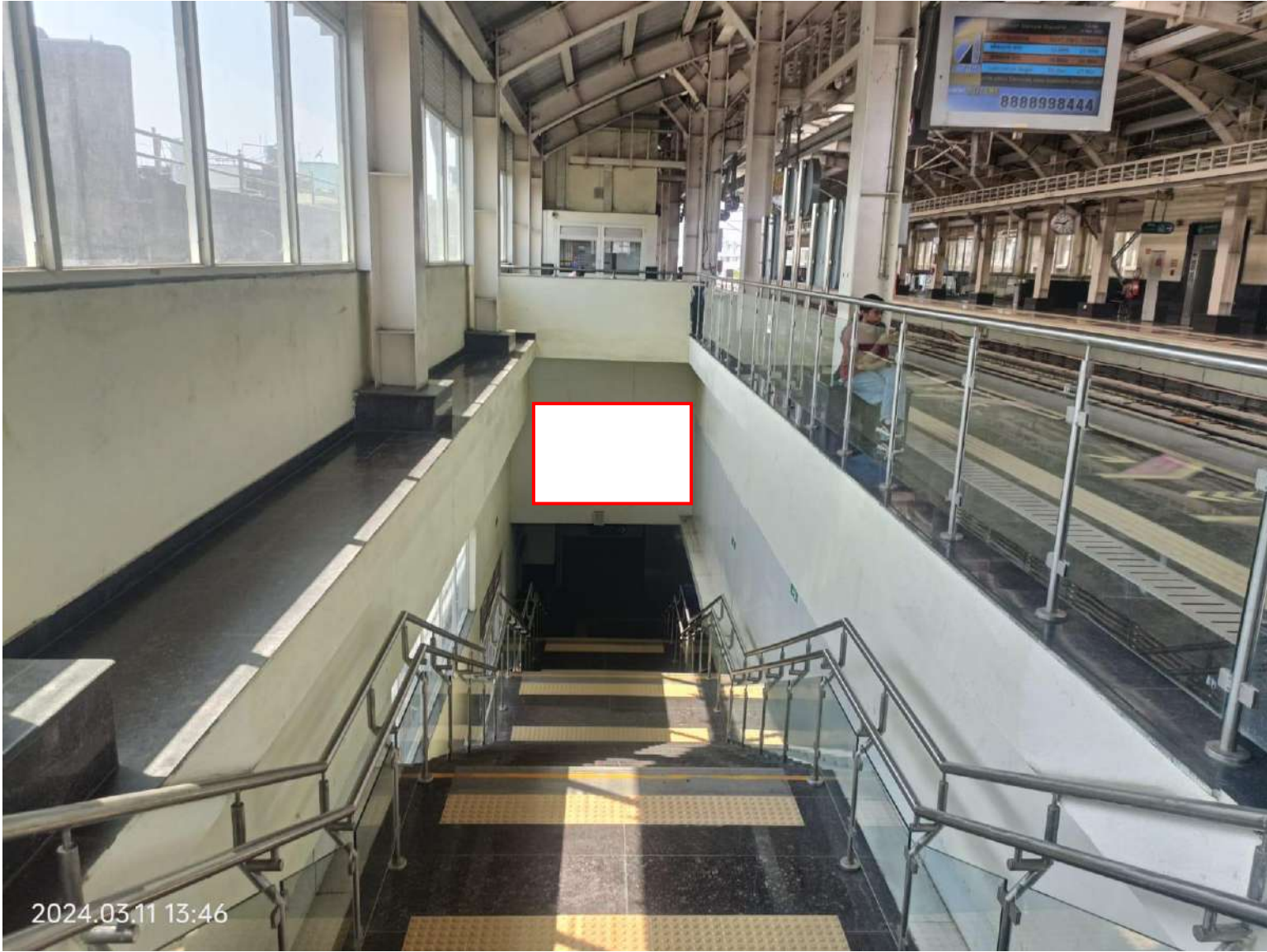
Dosar bhawan metro station platform 2 staircase upper Wall 8x5 a
