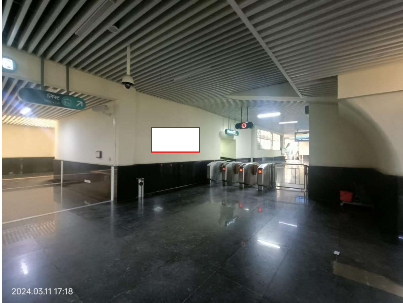
Rachna ring road metro station concourse 8x5
