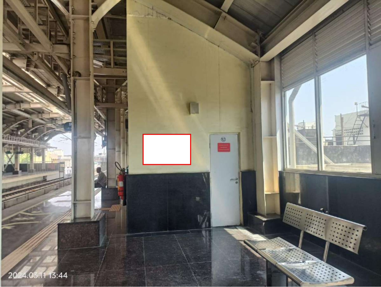
Dosar bhawan metro station platform 2 escalator side wall bench 5x8
