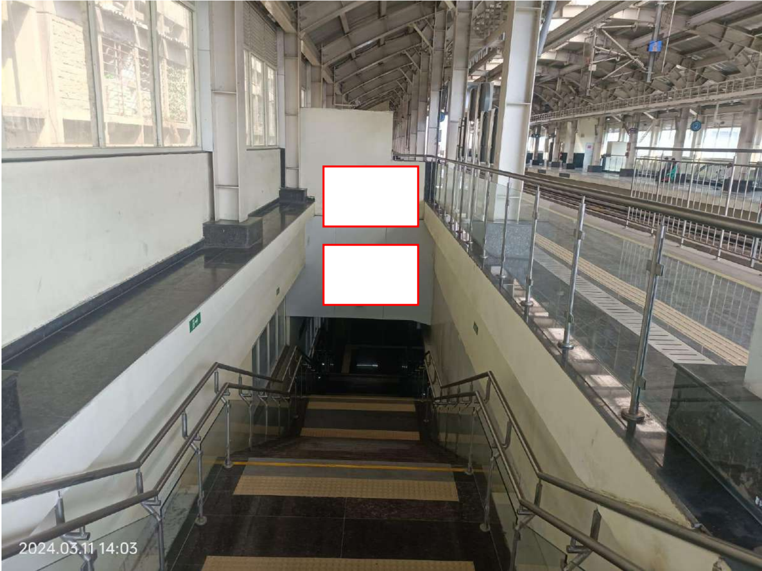
Dosar bhawan metro station platform 1 staircase upper Wall 8x5 (Qty 2)
