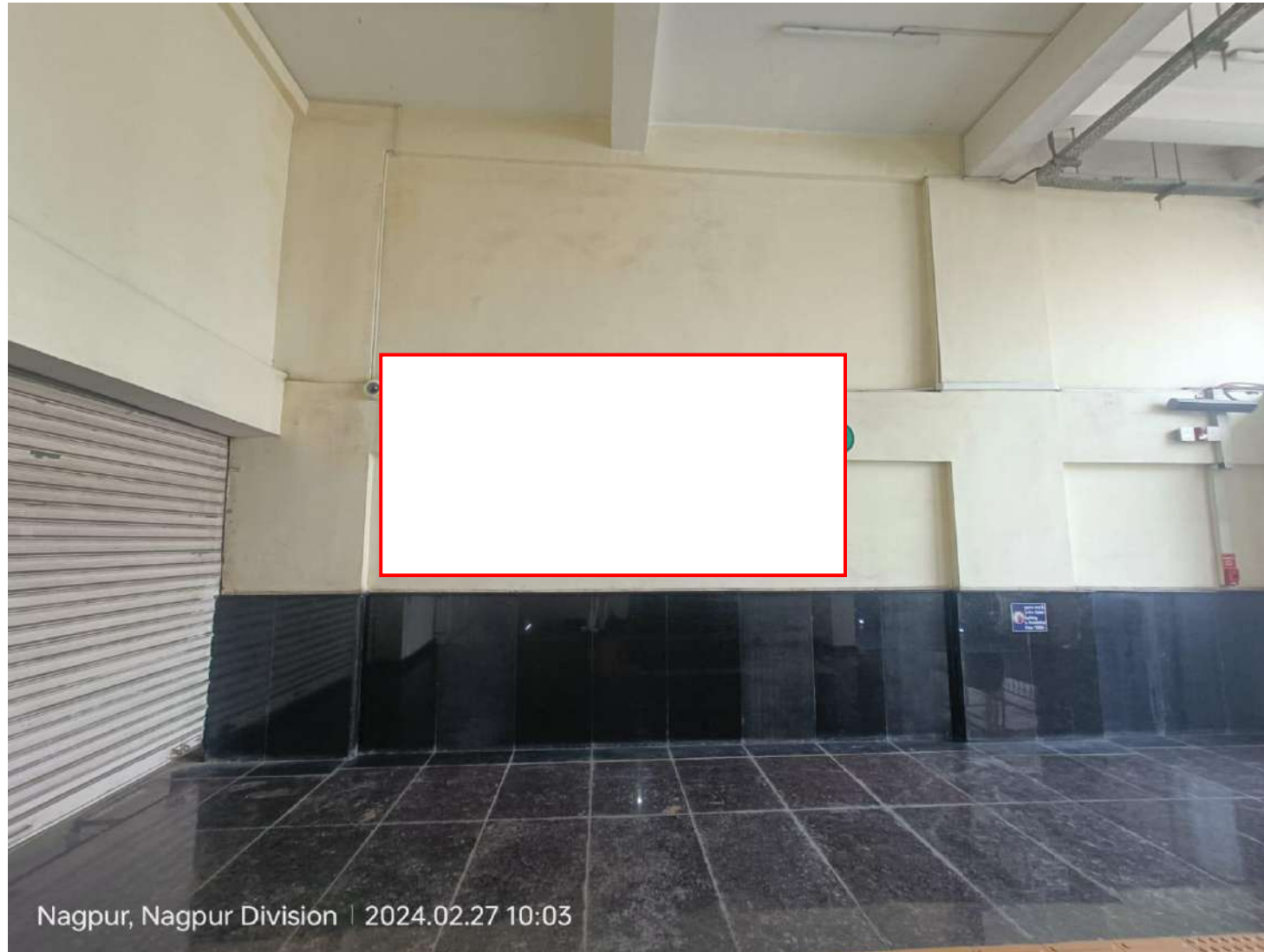
Prajapati nagar metro station staircase front wall 8x5
