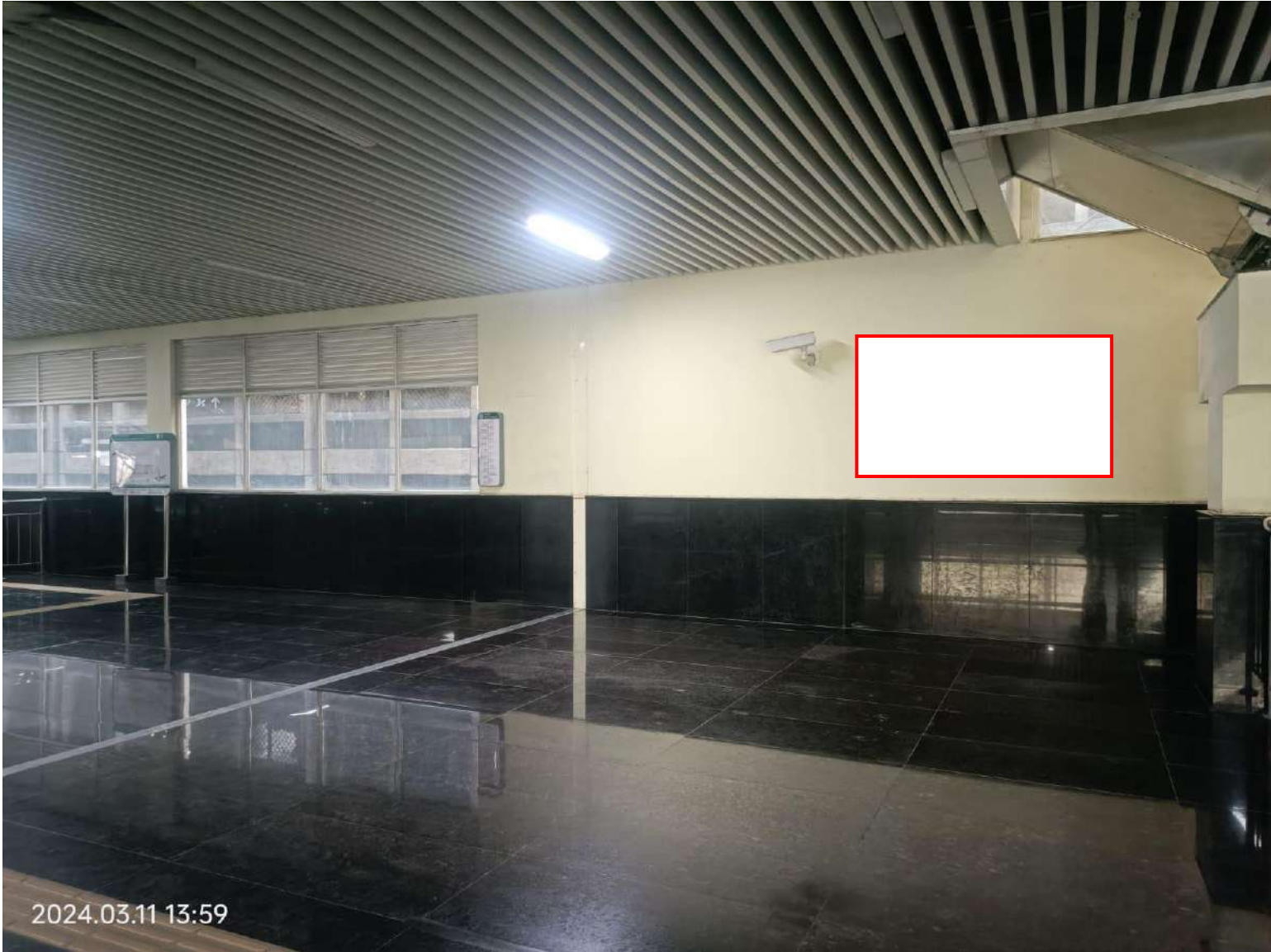
Dosar bhawan metro station concourse escalator done' wall 8x5
