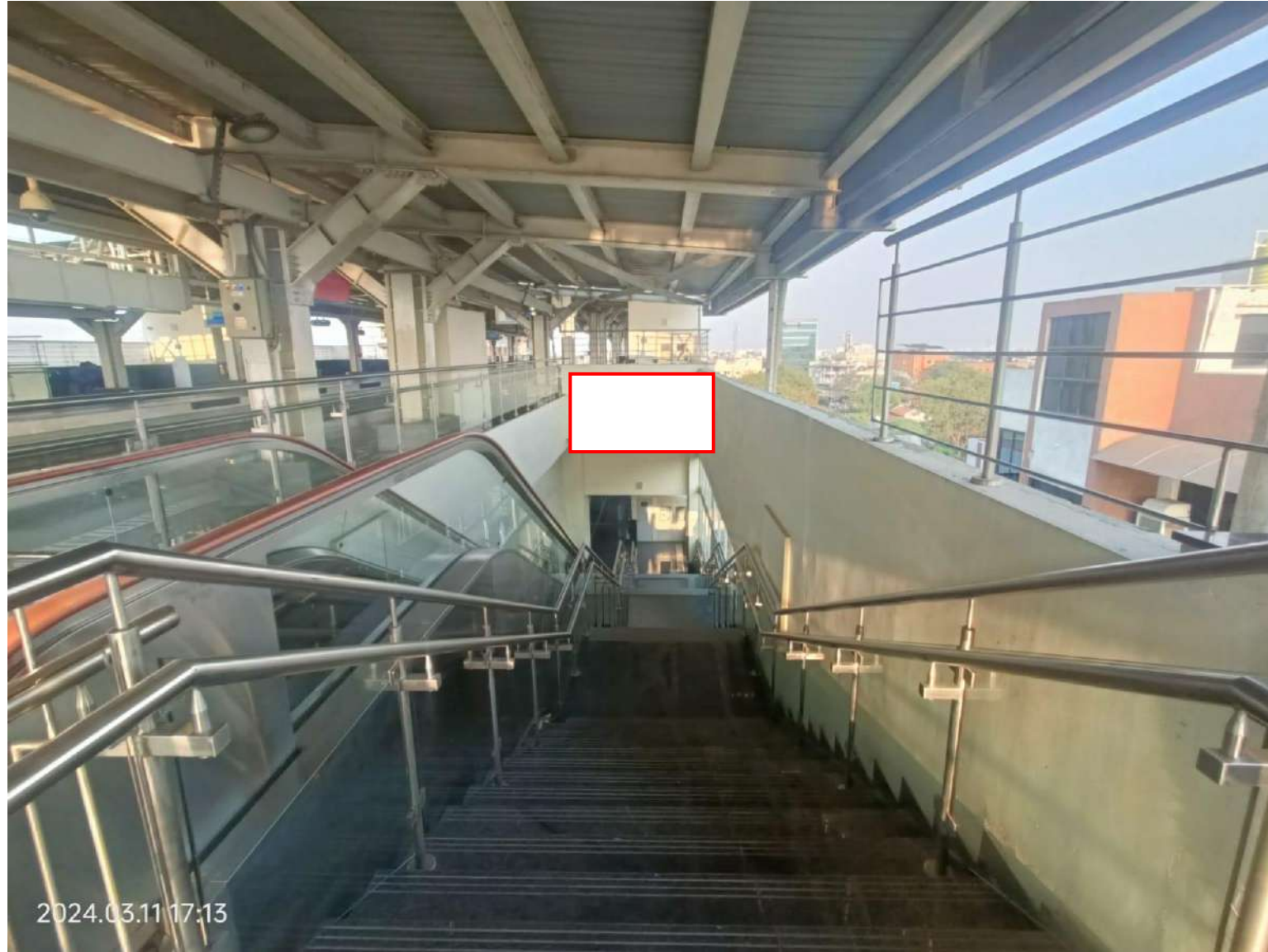
Rachna ring road metro station platform 2 escalator upper Wall 8x5
