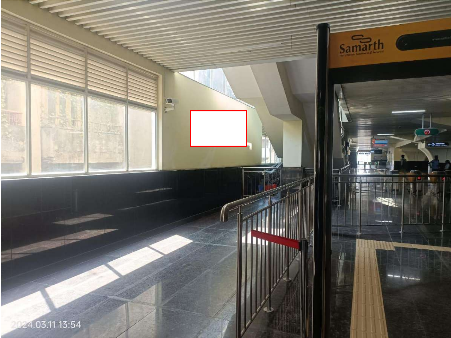
Dosar bhawan metro station entry concourse area front of ticket counter 8x5
