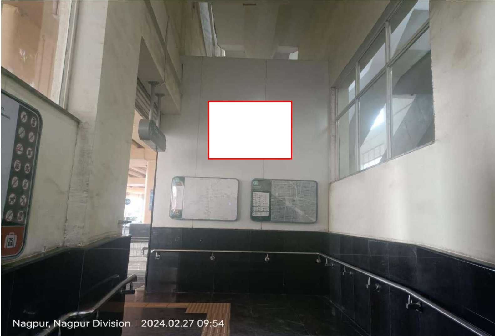
Prajapati nagar metro station entry lift front wall 8x5
