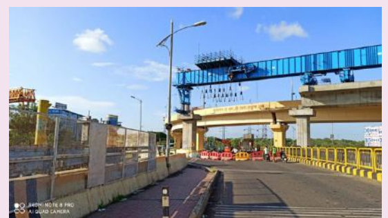
Erection of Last segment of Span 150-151 for Viaduct of Reach-1
